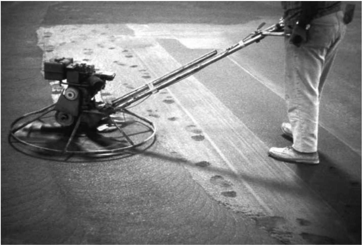
Power floating a screed.
