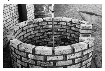
Although this takes time to set up, it makes accurate brick laying much quicker. (See photograph above right.) Unless the base will be plastered, a pointing tool is now used to finish the mortar between the bricks. To improve bond between bricks and mortar and make brick laying easier, clay bricks should be pre-soaked. If 'cement bricks' are used for the base, they should be laid dry.
