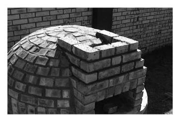
The chimney is constructed by building up above the oven door and over the top of the oven dome. Two low parallel 'walls' form the sides of the chimney. The side walls extend over the top of the dome.
