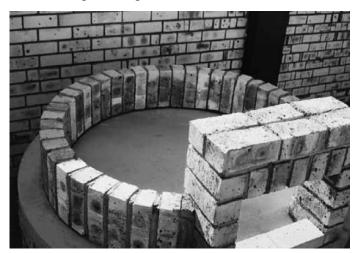
Lay a course of soldier bricks (bricks built up on end) to form the base of the dome. Use the 1,4 m circle as a guide to mark the position of the outside surface of this course of bricks. Allow the mortar to set and gain strength for at least 24 hours before any further work is done.
