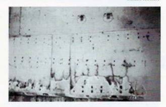
surface of the concrete member. Otherwise, cracking may occur. This is objectionable on aesthetic grounds if the concrete surface is apparent, and on durability grounds if an attacking medium can penetrate through the cracks toward the reinforcement.
