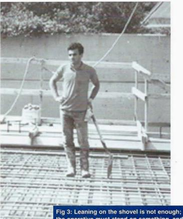
Fig 3: Leaning on the shovel is not enough; the operative must stand on something, and reinforcing steel must be supported.
