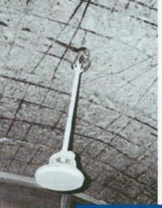
Fig 1: Catastrophic delamination of soffit of a slab due to inadequate cover for extreme exposure conditions
