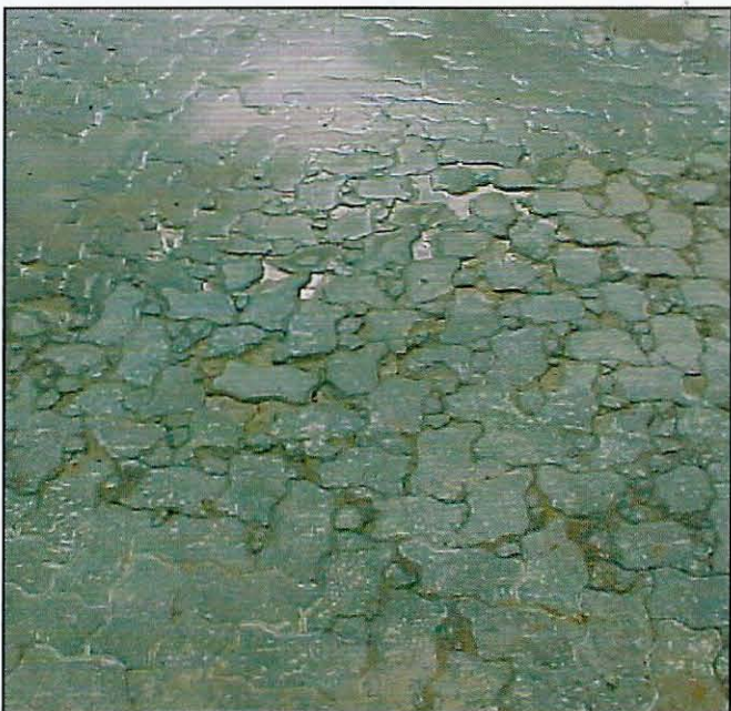
Figure 3. Deteriorated block paving at Belle Ombre bus depot
