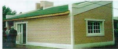
Figure 13. Housing unit utilising dry-stack earth-block units.
