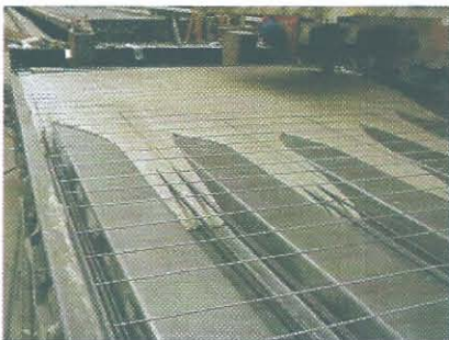
Figure 1: Self compacting concrete does not need any external vibration for full compaction and filling of formwork
