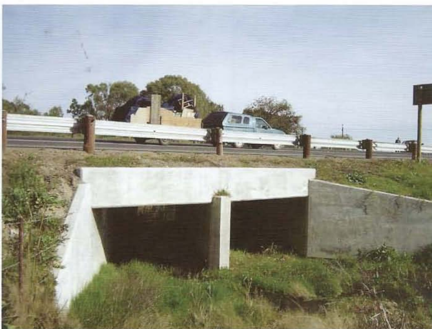
Fig. 5: Repaired culvert in Cape Town
