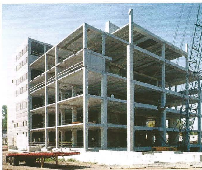
Figure 3: Example of skeletal frame design with internal columns (Spancrete, USA).
