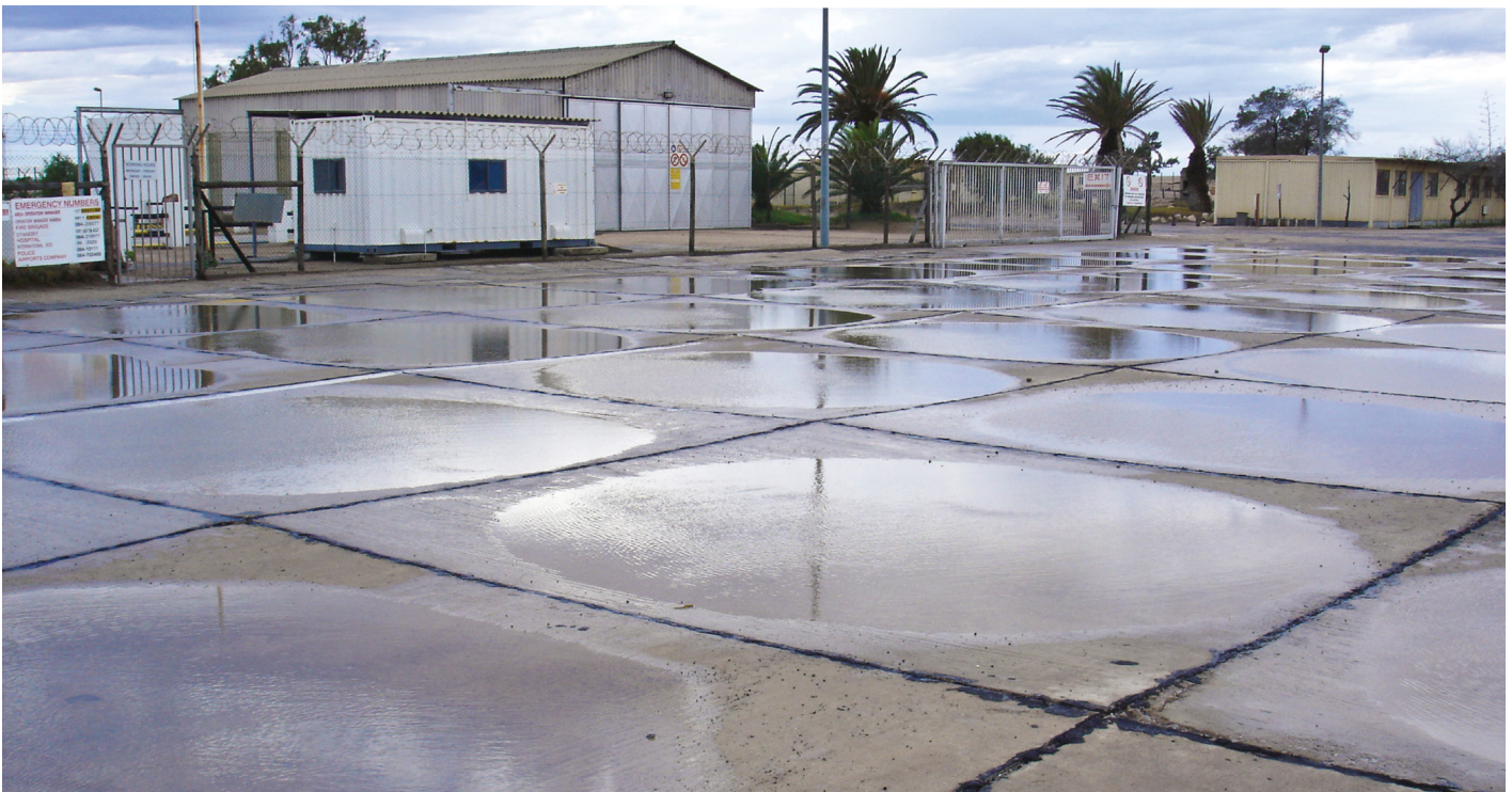
Figure 2: An excellent example of extreme curling of concrete panels in the apron at Walvis Bay Airport after a rare high rainfall event; note the extreme lifting of corners and perimeter edges relative to the centre (Photo: Roderick Rankine)
