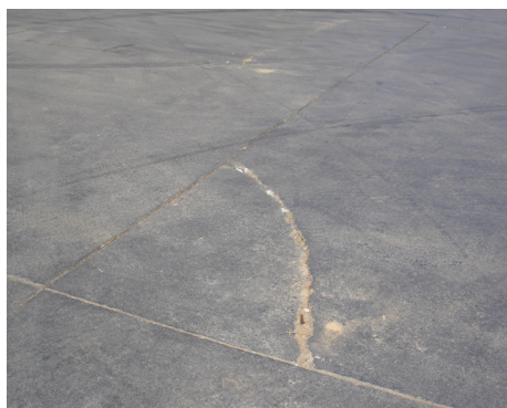
Figure 3: Corner cracking of curled slabs under heavy traffic is a common symptom of curled ground slabs, particularly if load-transfer is absent or compromised; the elevated corner essentially becomes an unpropped unreinforced cantilever
