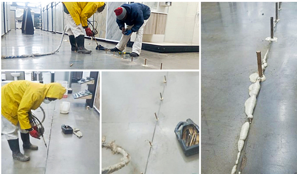
Figure 6: Joint filling and rocking slab stabilisation by injection of polyurethane expanding foam into the void beneath saw-cut contraction joints at regular intervals; as the foam expands, it rises and infiltrates the joints from the bottom up (Photo: Chris Howes Construction)
