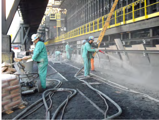
Dry-mix shotcrete Today
