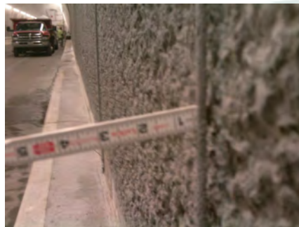
Prepared substrate ready for application of flashcoat.
