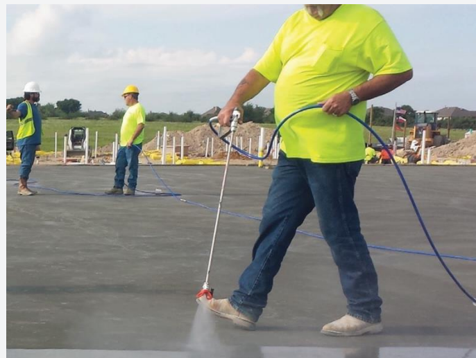
Colloidal silica applied to a concrete surface
